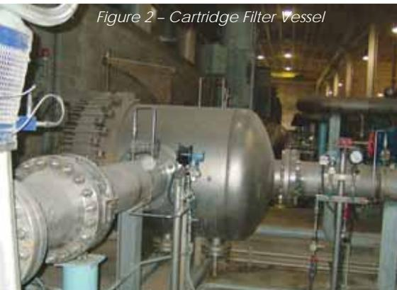
Figure 2 – Cartridge Filter Vessel
